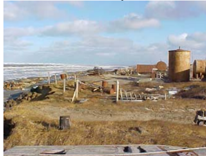
“Nayokpuk General Store’s Bulk Fuel Farm”
