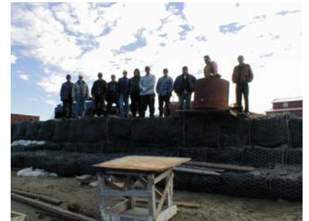
“Summer 2001 gabion construction crew”
