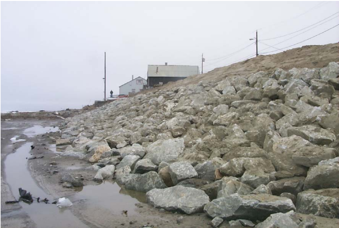
Final work Kaverak Seawall Project – 450'
